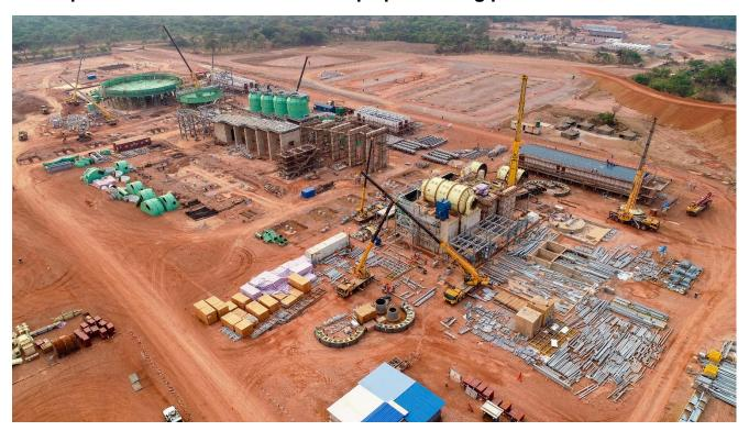
Flotation cells, manufactured by Outotec, in Finland and South Africa, installed at Kakula's initial 3.8-Mtpa processing plant.
