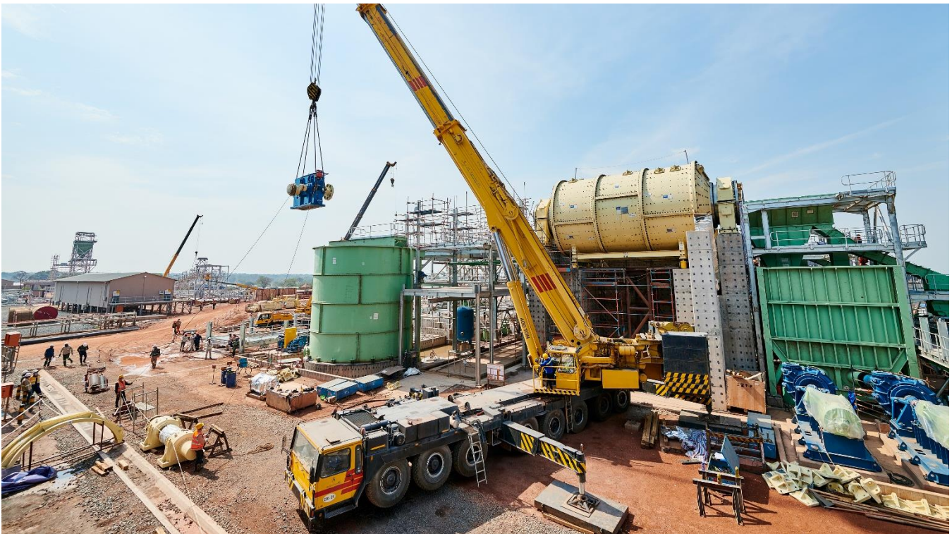
Lifting the reducer gear box assembly for the Phase 2 secondary ball mill.
