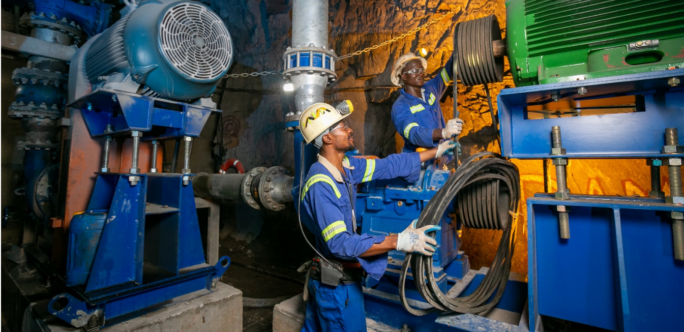
Leandro Sanga, Underground Supervisor (left), and Mack Mwambu, underground worker, installing drive belts for a water pump at the Kakula Mine.
