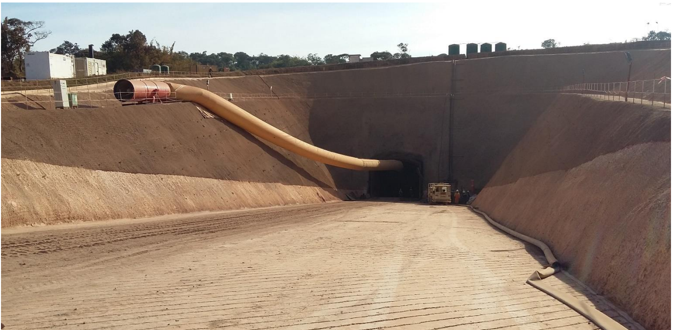
Figure 11: Kakula's southern box cut and portal entrance to the decline.
