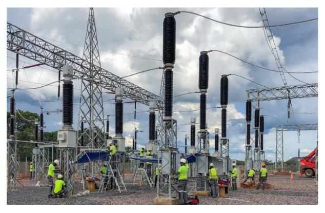
Kakula's 220-kilovolt main substation and power line connecting to the grid.
