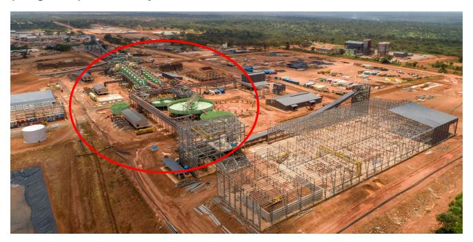
Second stage (C2) commissioning at Kamoa-Kakula's Phase 1 ball mills (in yellow) and the concrete foundations for the second set of ball mills for the Phase 2 concentrator (foreground), are underway.
