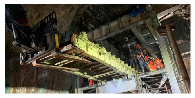
Kakula's underground construction team nearing completion of the bottom structure of the east tip, part of the underground ore handling system at Kakula.
