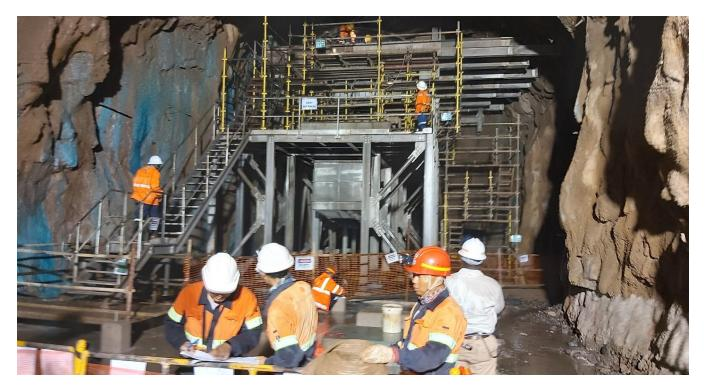
Raise boring machine breaks through to surface, marking the completion of reaming the 5.5-metre diameter Ventilation Shaft 2 at the Kakula Mine.
