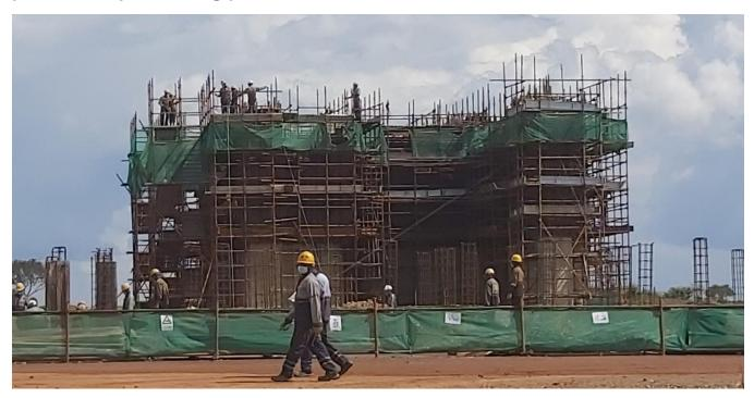
Pouring the concrete foundations for the processing plant's concentrate thickener.
