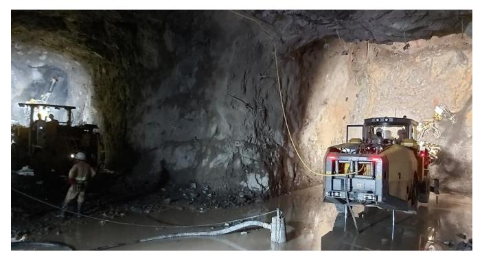
Construction crew extending the wall at Kakula's main underground water storage dam.
