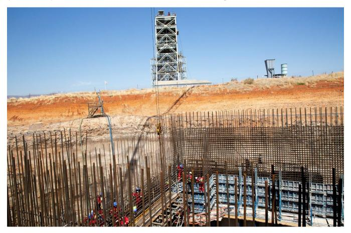
Platreef's Shaft 2 will have a finished and concrete-lined internal diameter of 10 metres and be sunk to a planned, final depth of 1,104 metres below surface.
