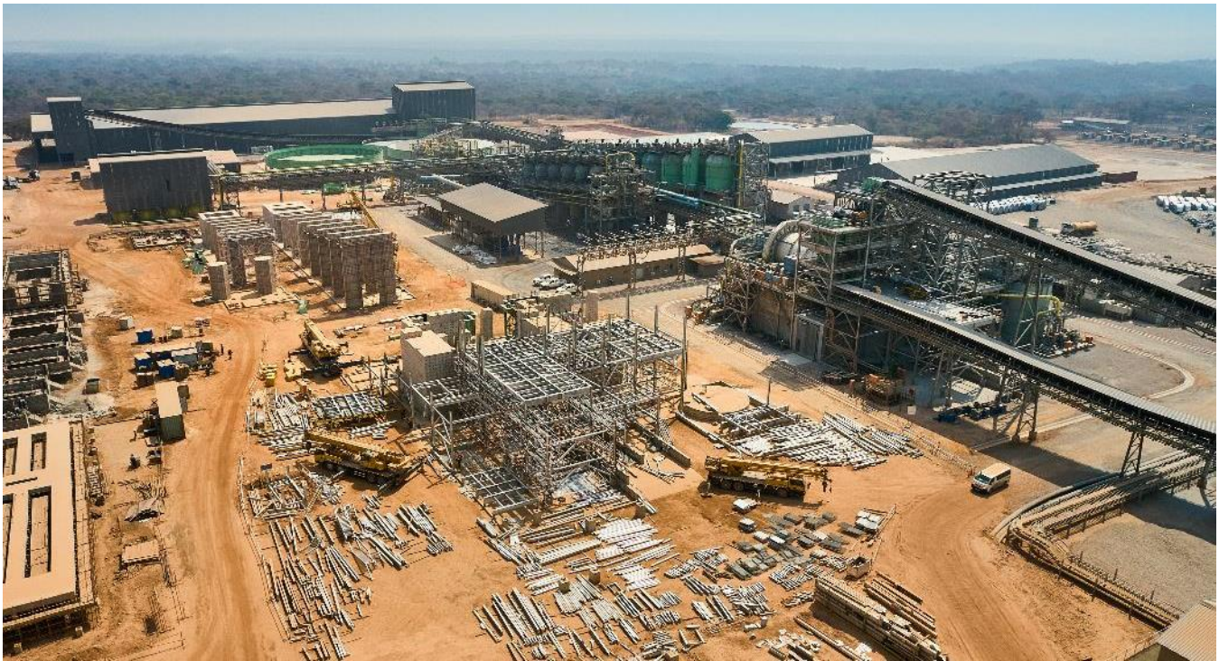
Construction of the Phase 2 tailings thickener is nearing completion.
