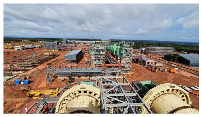
Kakula's Phase 1 backfill plant is nearing completion. Approximately one half of the mine's tailings will be sent back underground as paste backfill to help support mined-out areas.
