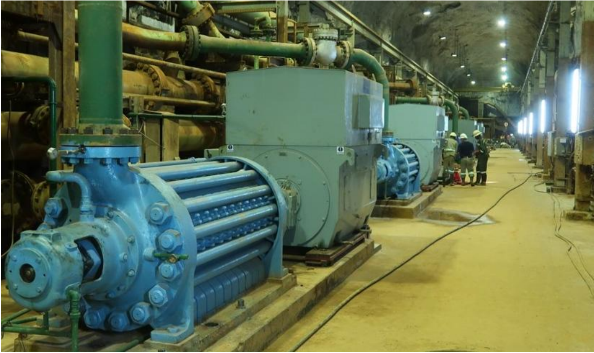
Figure 4. New high-capacity water pumps at Kipushi's 1,200-metre level.
