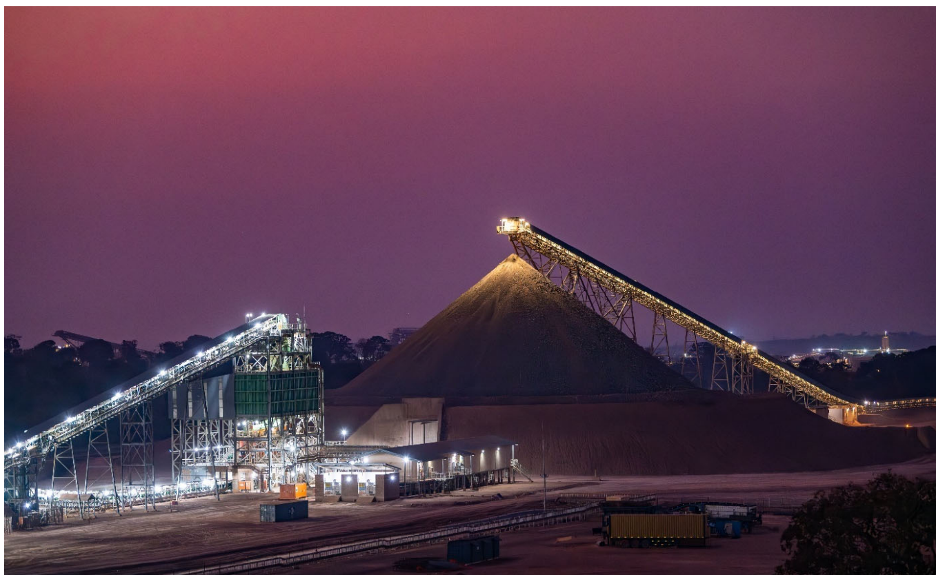
Photo: The Phase 3 concentrator run-of-mine stockpile. As of June 30, 2024, a total of 2.51 million tonnes of ore at an average grade of 2.85%, containing over 70,000 tonnes of copper, was stored in stockpiles near the Phase 3 concentrator.
