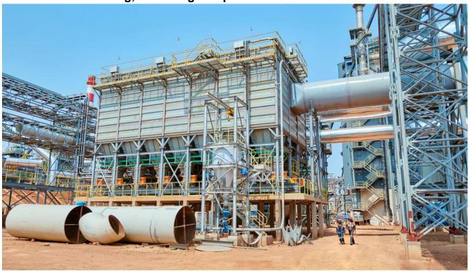
Waste heat captured from the furnace building is recycled to generate 8 megawatts of electricity, which will be used as supplementary power for the smelter operations.
