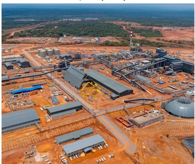
The smelter construction site includes a milling and flotation plant designed to reprocess slag generated by the smelter, taking overall recoveries to approximately 98%.
