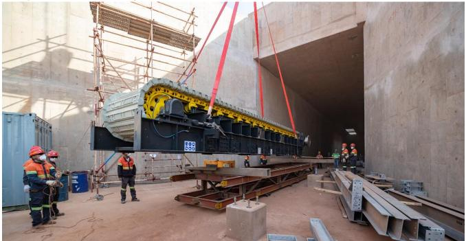
Steel erection of Kamoa-Kakula's direct-to-blister flash furnace and the electric slag cleaning furnace. The 500,000 tonnes-per-annum copper smelter, will be the largest in Africa and one of the largest in the world.
