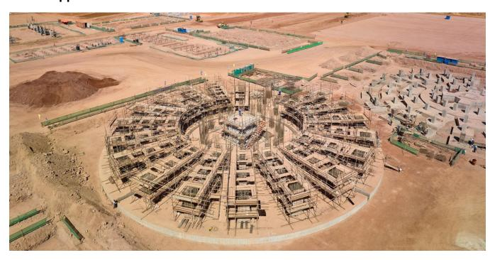
Steel erection of Kamoa-Kakula's direct-to-blister flash furnace and the electric slag cleaning furnace. Overall smelter construction is now approximately 50% complete. Fabrication of the anode furnaces, ball mill and SAG mill, also manufactured by CITIC Heavy Industries, is complete with shipping expected imminently.
