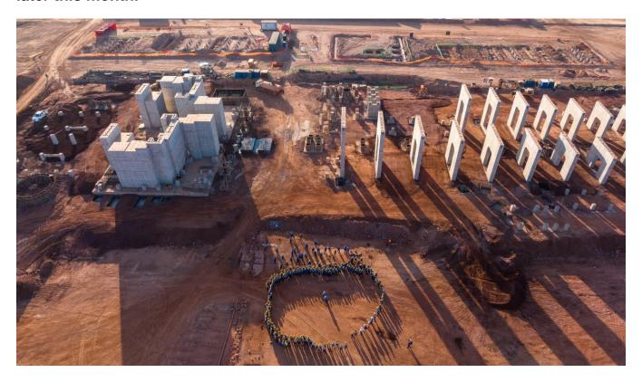
Concrete foundations for the Phase 3 concentrator tailings thickener. Over 60% of concrete has been poured to date and approximately 6,000 tonnes of the required 7,100 tonnes of structural steel have been fabricated, 50% of which has been shipped to site.
