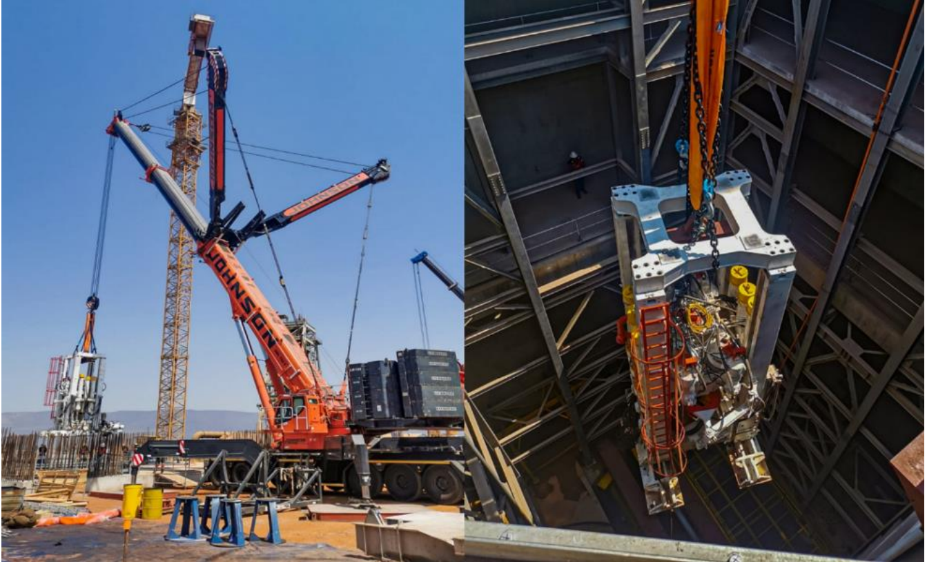
Shaft 2 raise-boring equipment being lowered into position.
