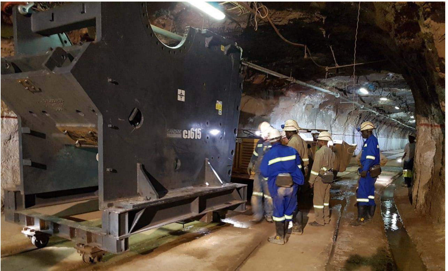
The main frame being transported to the 1,150-metre-level crusher chamber.
