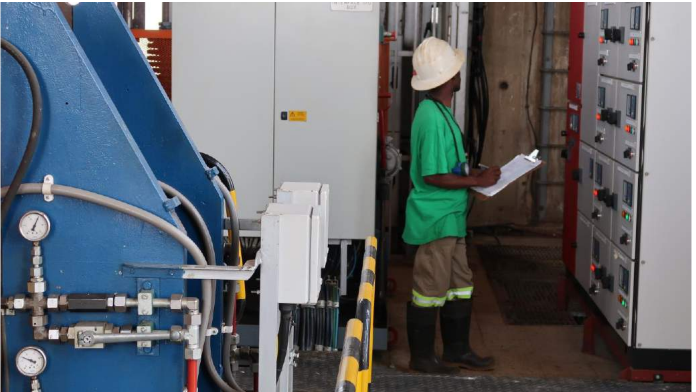
A new electrical subpanel for one of the winders.
