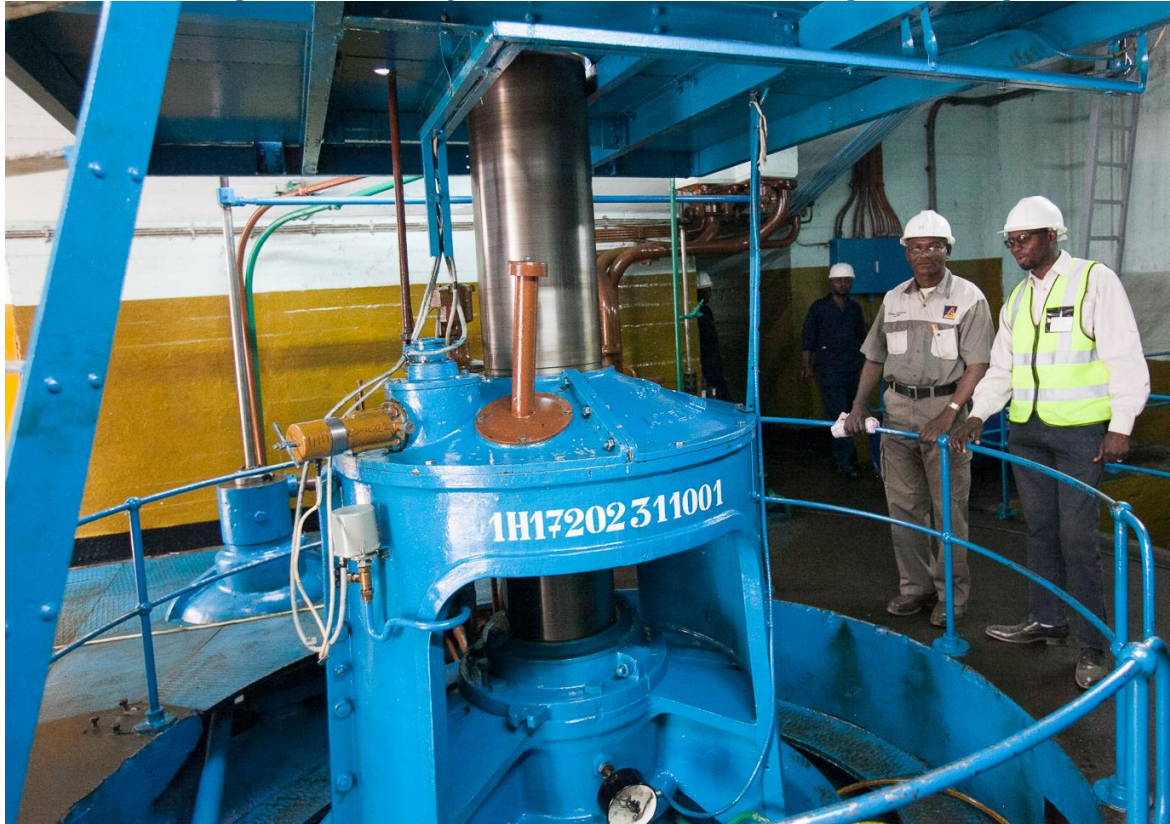
Photo 4. Reconditioned crane and new alternator at Mwadingusha.
