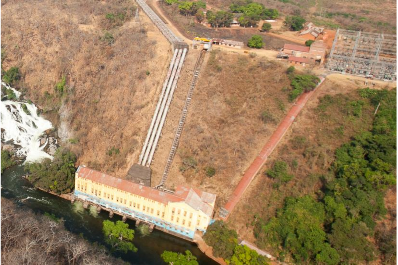
Photo 6. Mwadingusha hydropower plant and sub-station.
