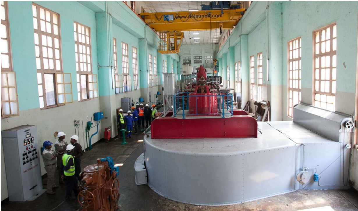
Photo 4. Reconditioned crane and new alternator at Mwadingusha.
