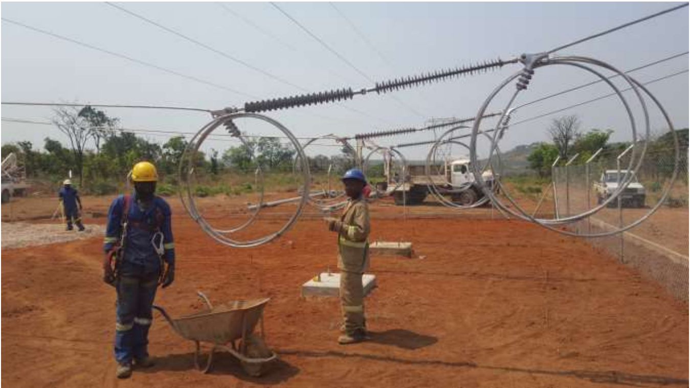
Figure 12. Workers installing a 120kV power line at the Kamoja Project.
