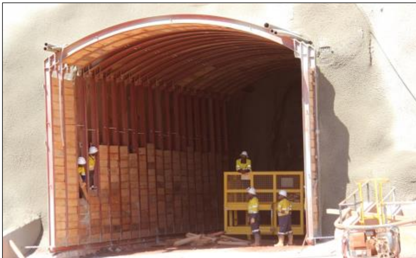
Figure 7. Conveyor decline sets.
