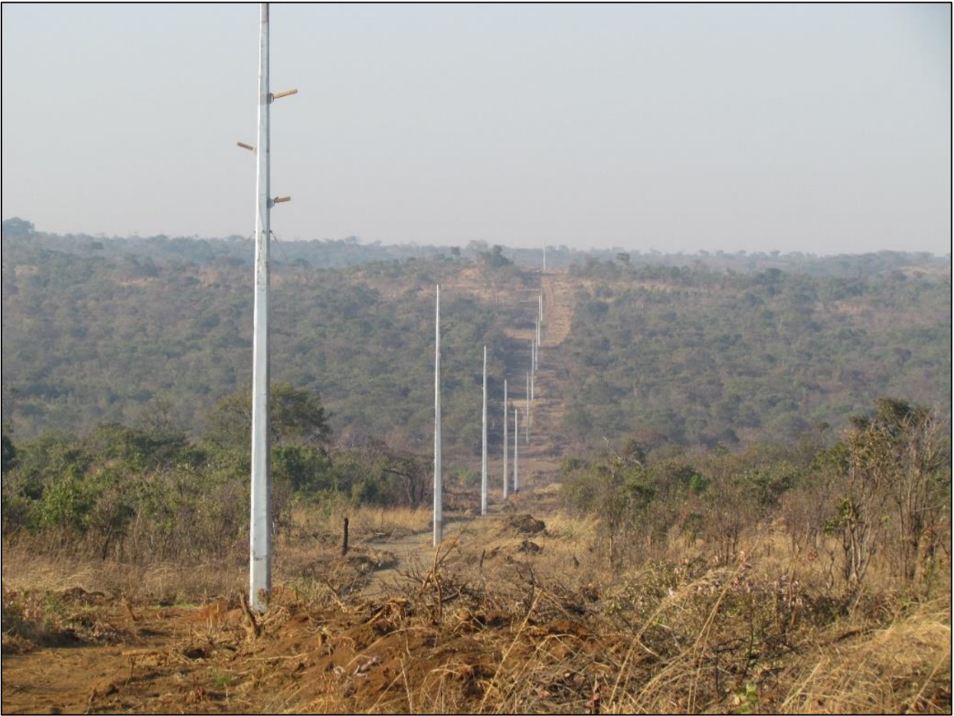
Figure 11. 120 kV power line under construction.
