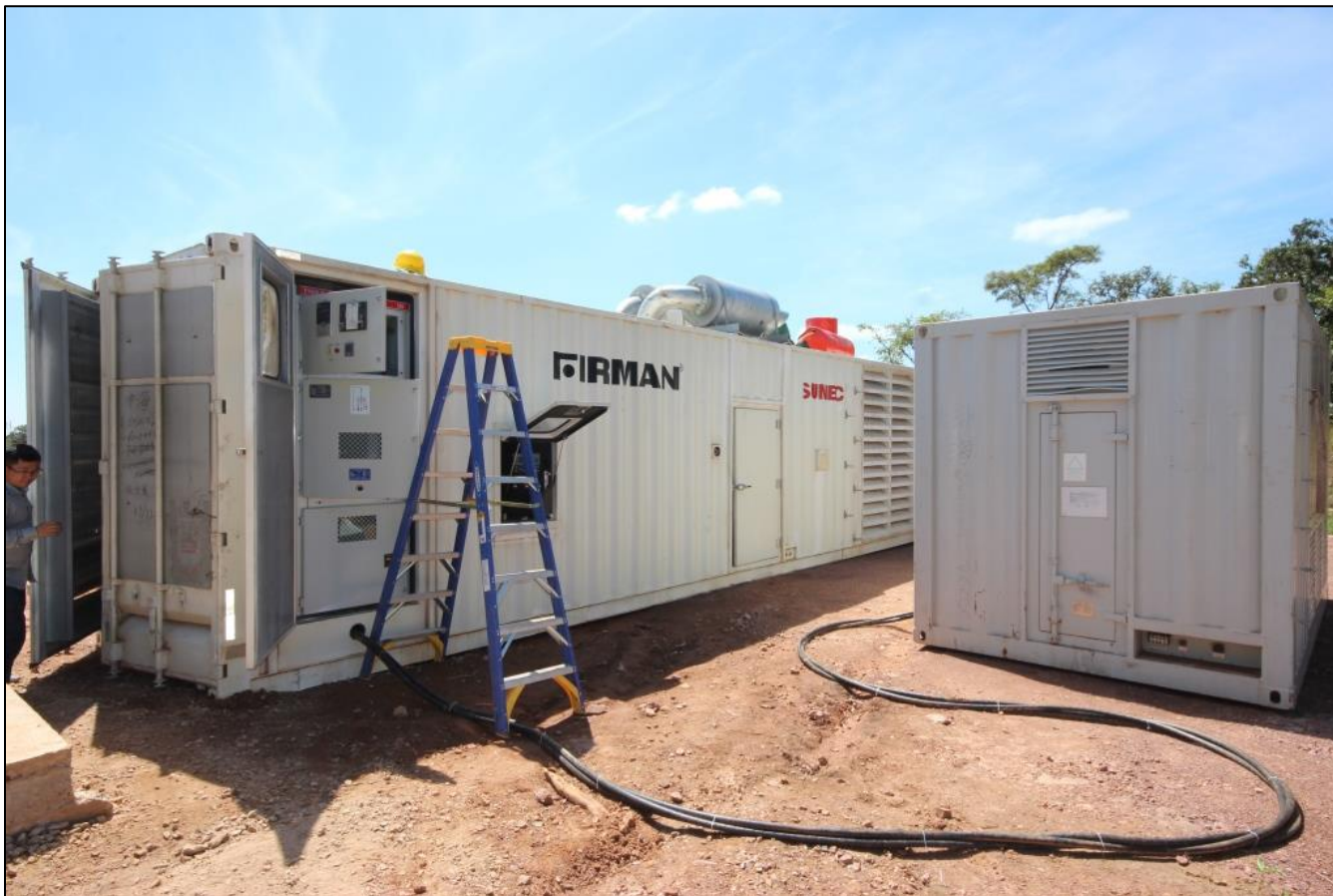
Figure 10. Sumec 2-MW generator being commissioned.
