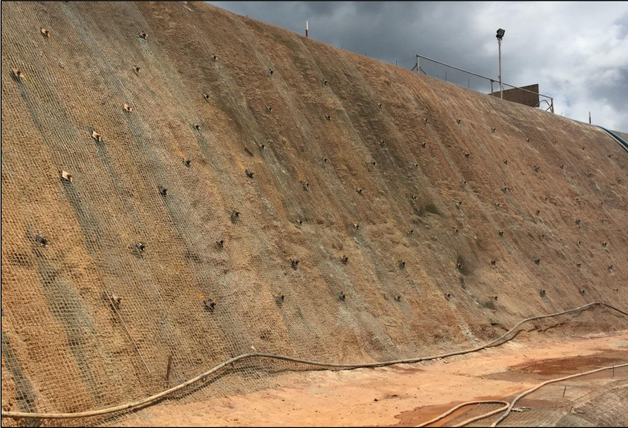
Shotcrete application on the bottom bench.
