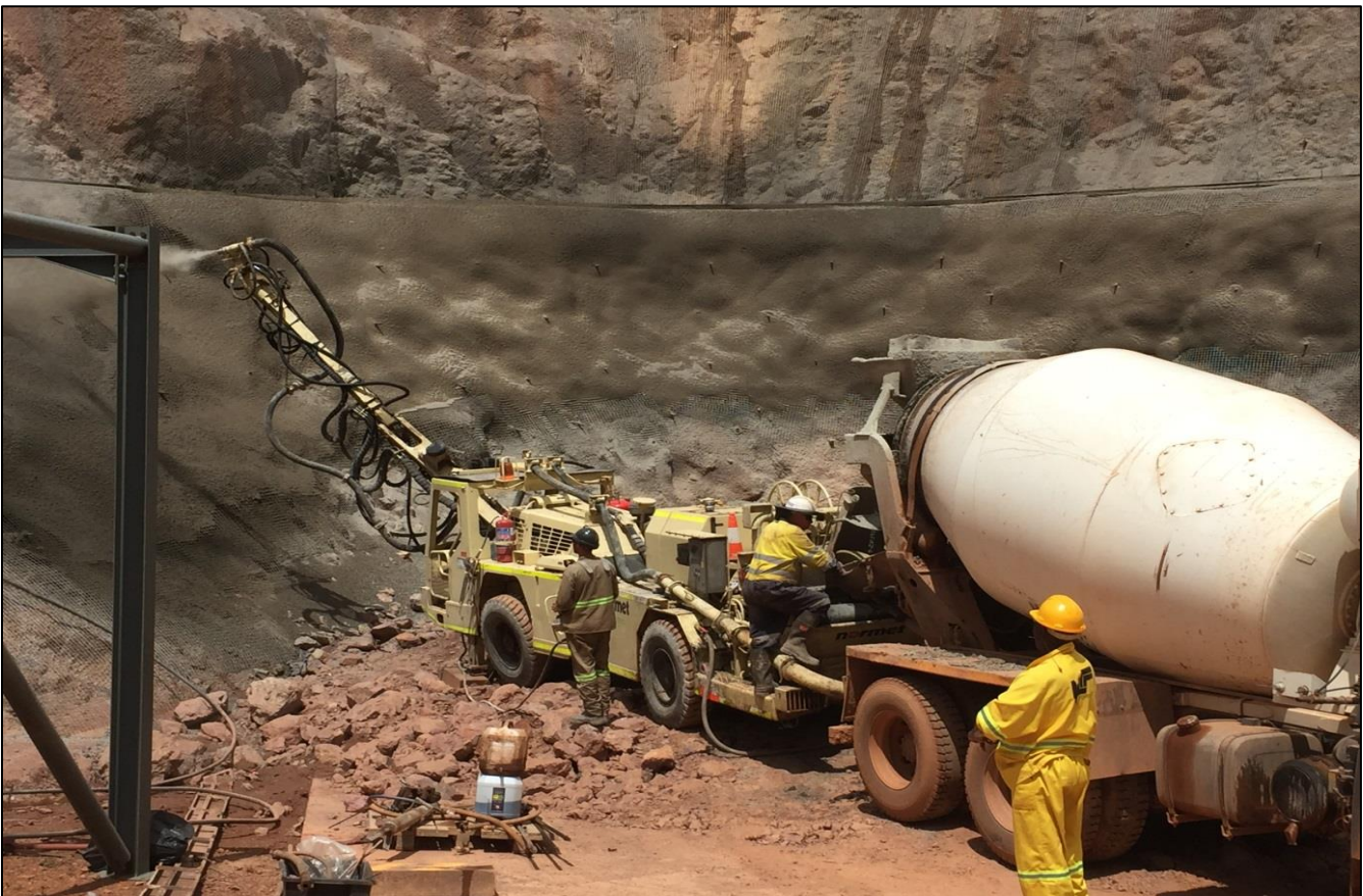
Shotcrete application on the bottom bench.
