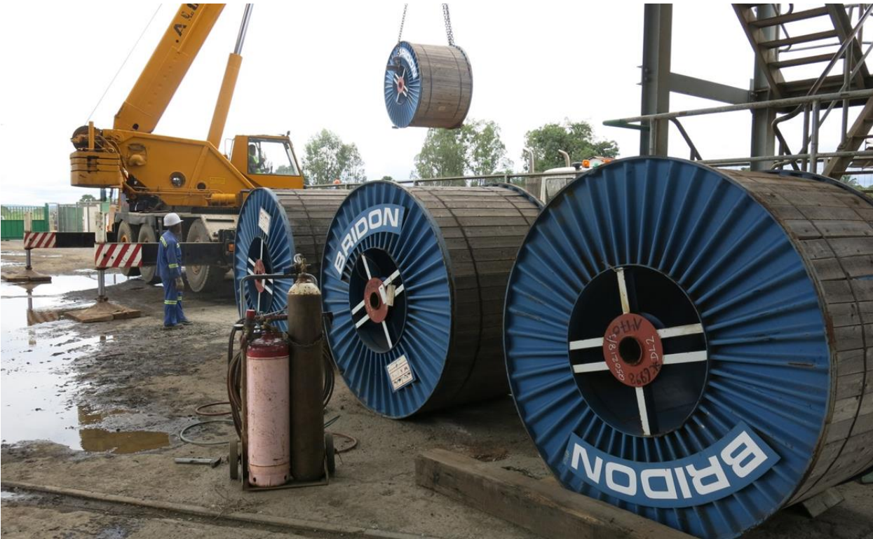
Figure 13: Off-loading new wire rope for the Shaft 5 hoist
