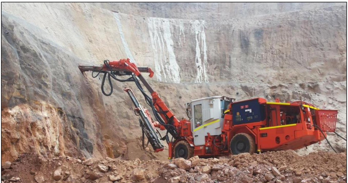
Figure 16: Drilling of anchor-bolt holes at the Kamoia box cut.
