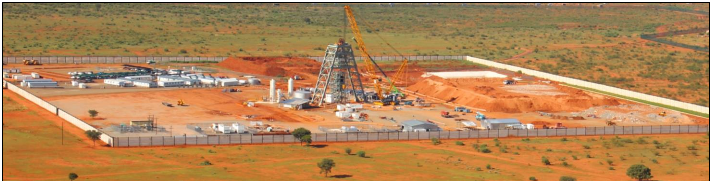
Figure 1: Aerial view of the Platreef Project site.
