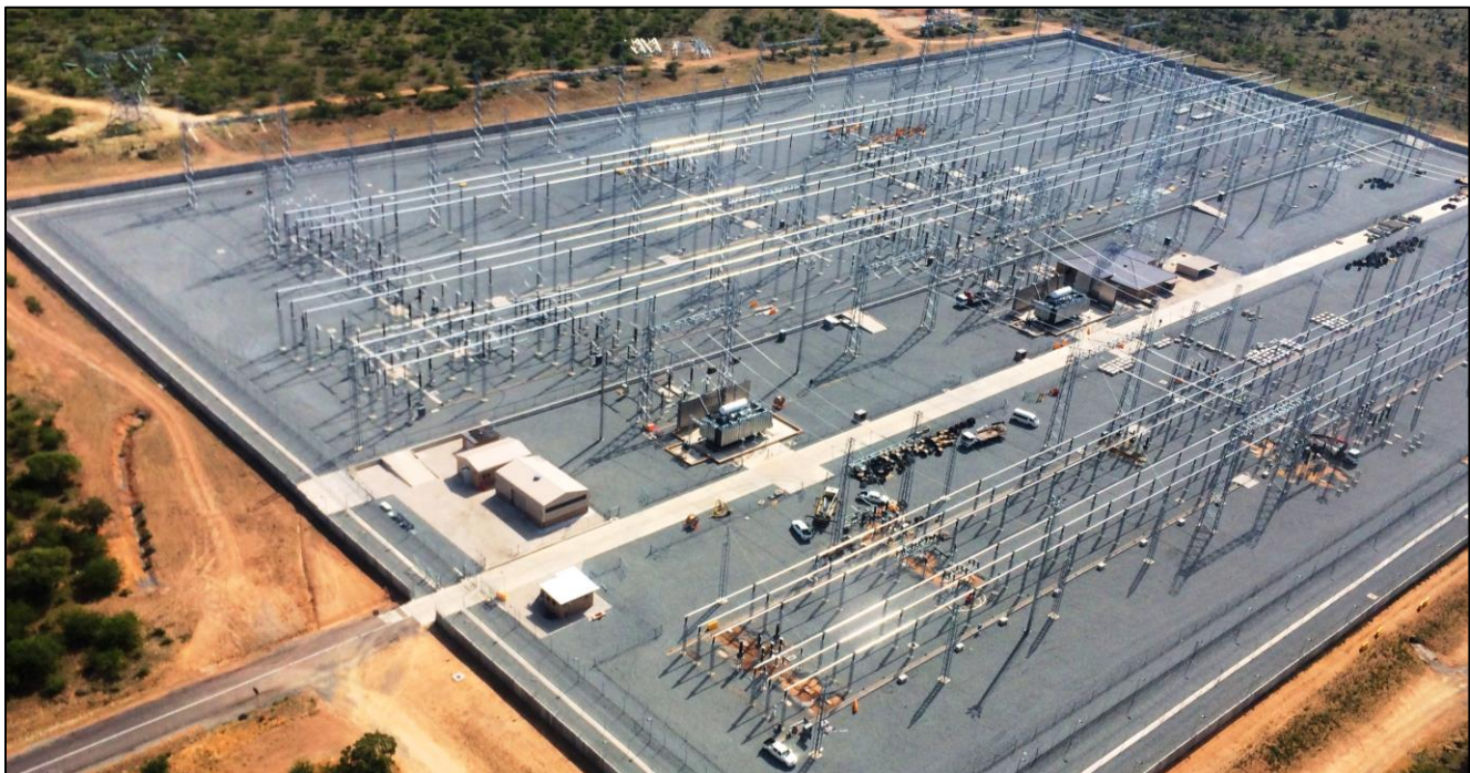
Figure 7: Construction of the Eskom Borutho substation.
