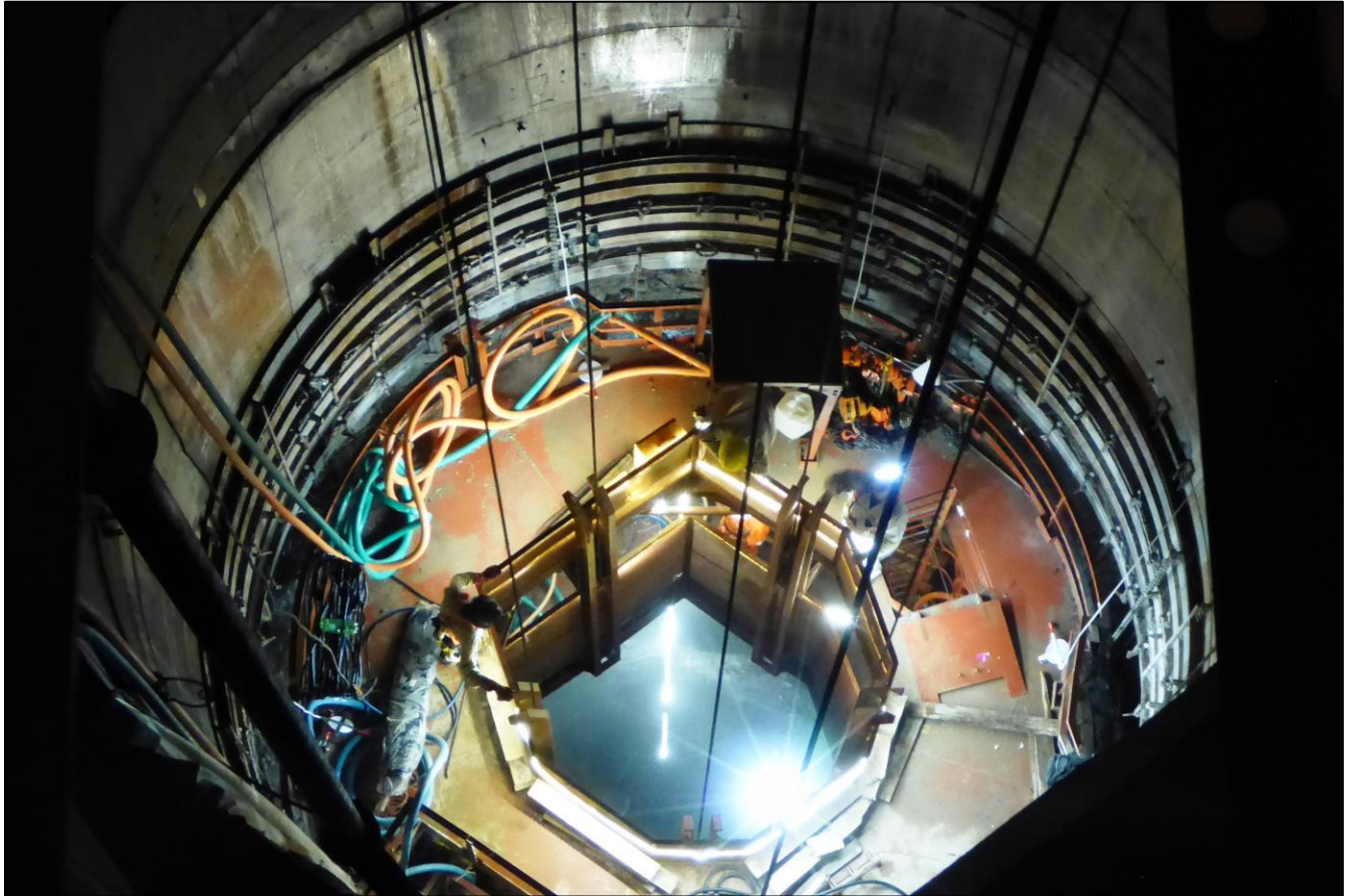
Figure 5: Internal view of shaft-sinking activities during the pre-sink phase.
