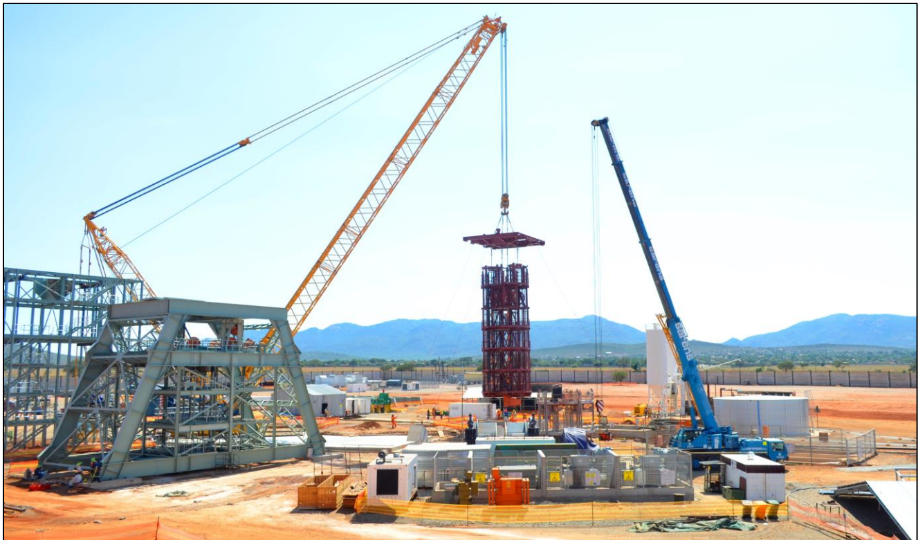
Figure 2: Lowering of the five-deck stage and bank steelwork into Shaft 1.
