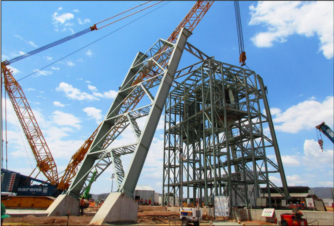
Figure 4: Shaft 1 main-sink headgear.
