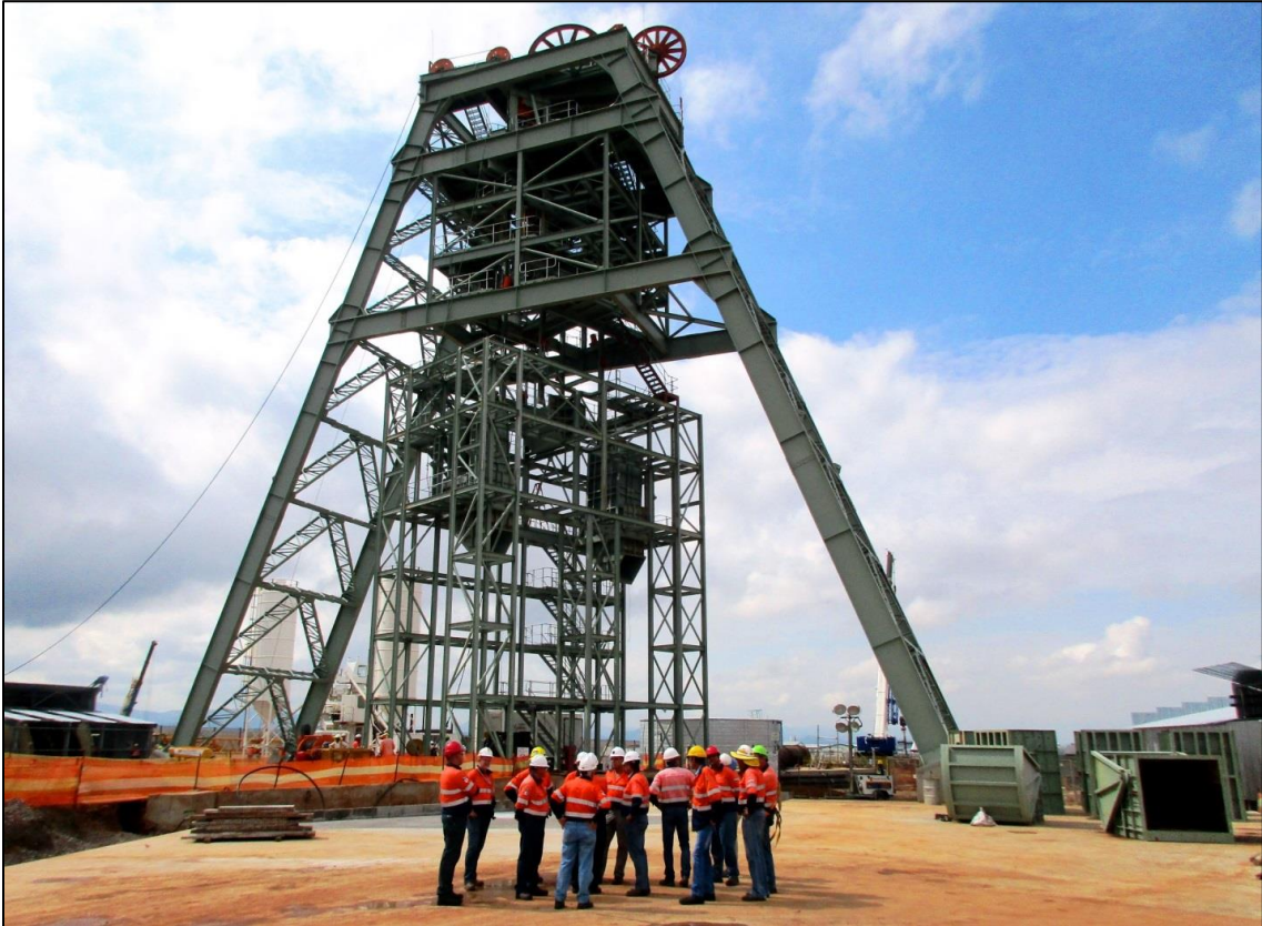
Figure 4: Shaft 1 main-sink headgear.
