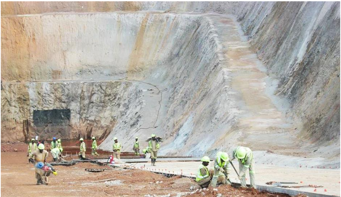
Figure 1: Completed box cut with access roadway under construction.
