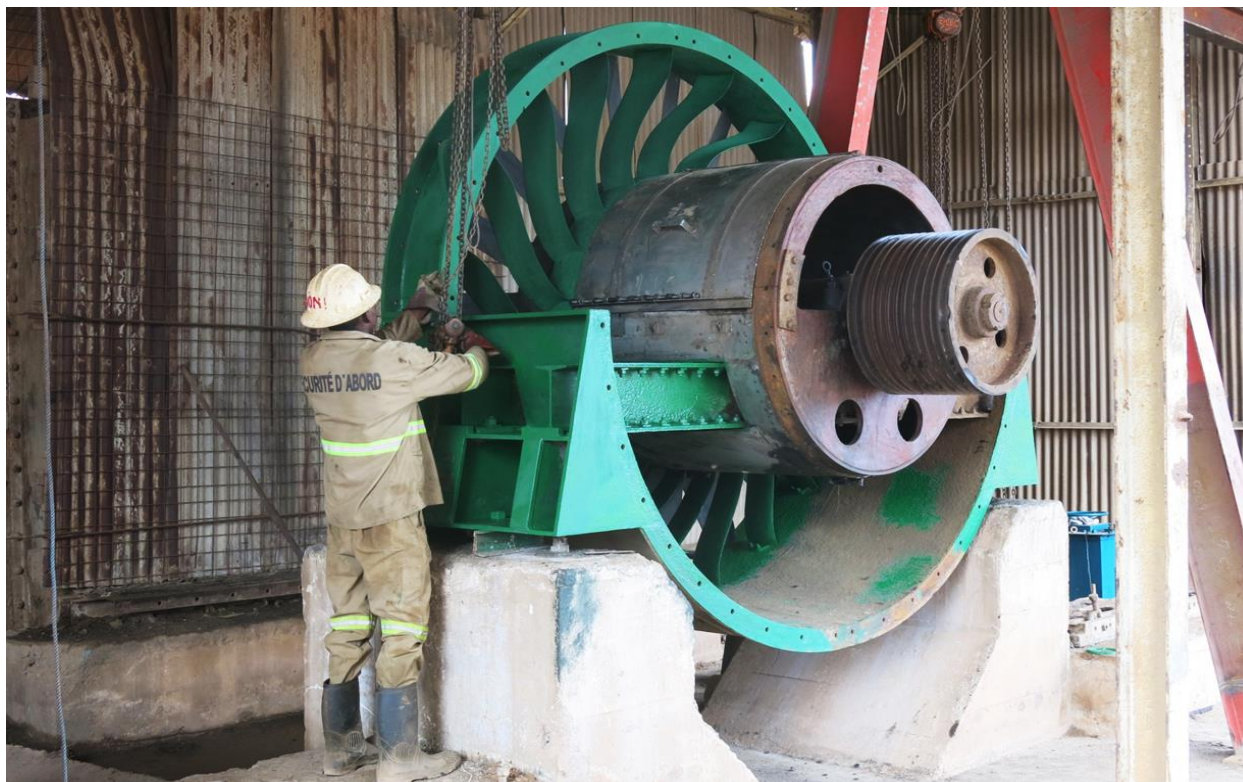
Figure 11: Ventilation shaft fan refurbishment.
