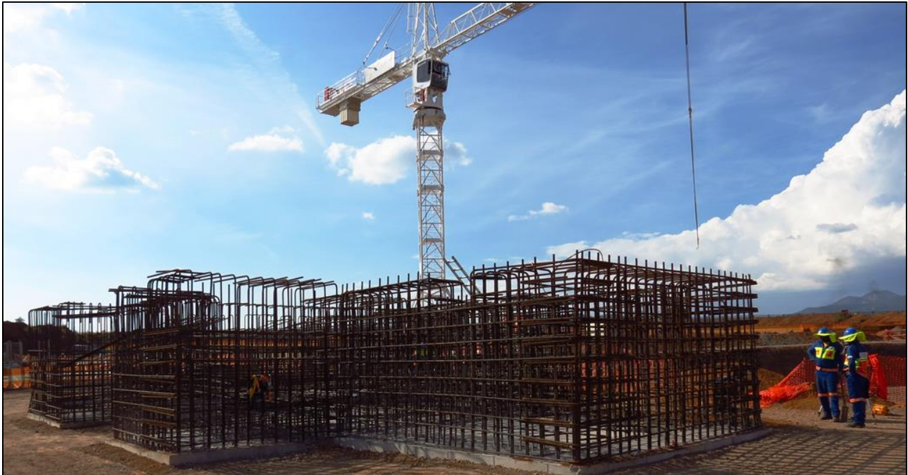
Figure 6: Construction of Shaft 1 kibble winder foundation.
