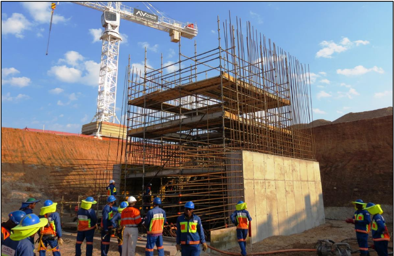
Figure 5: Construction of Shaft 1 collar, May 8, 2015.
