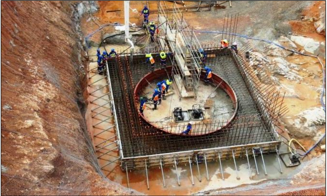
Figure 5: Construction of Shaft 1 collar, May 8, 2015.
