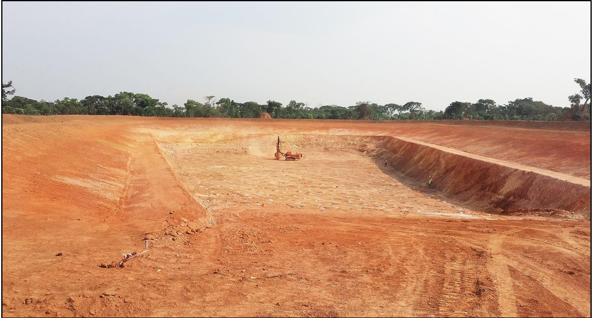
Figure 3: Blasting at box-cut site, September 20, 2014.
