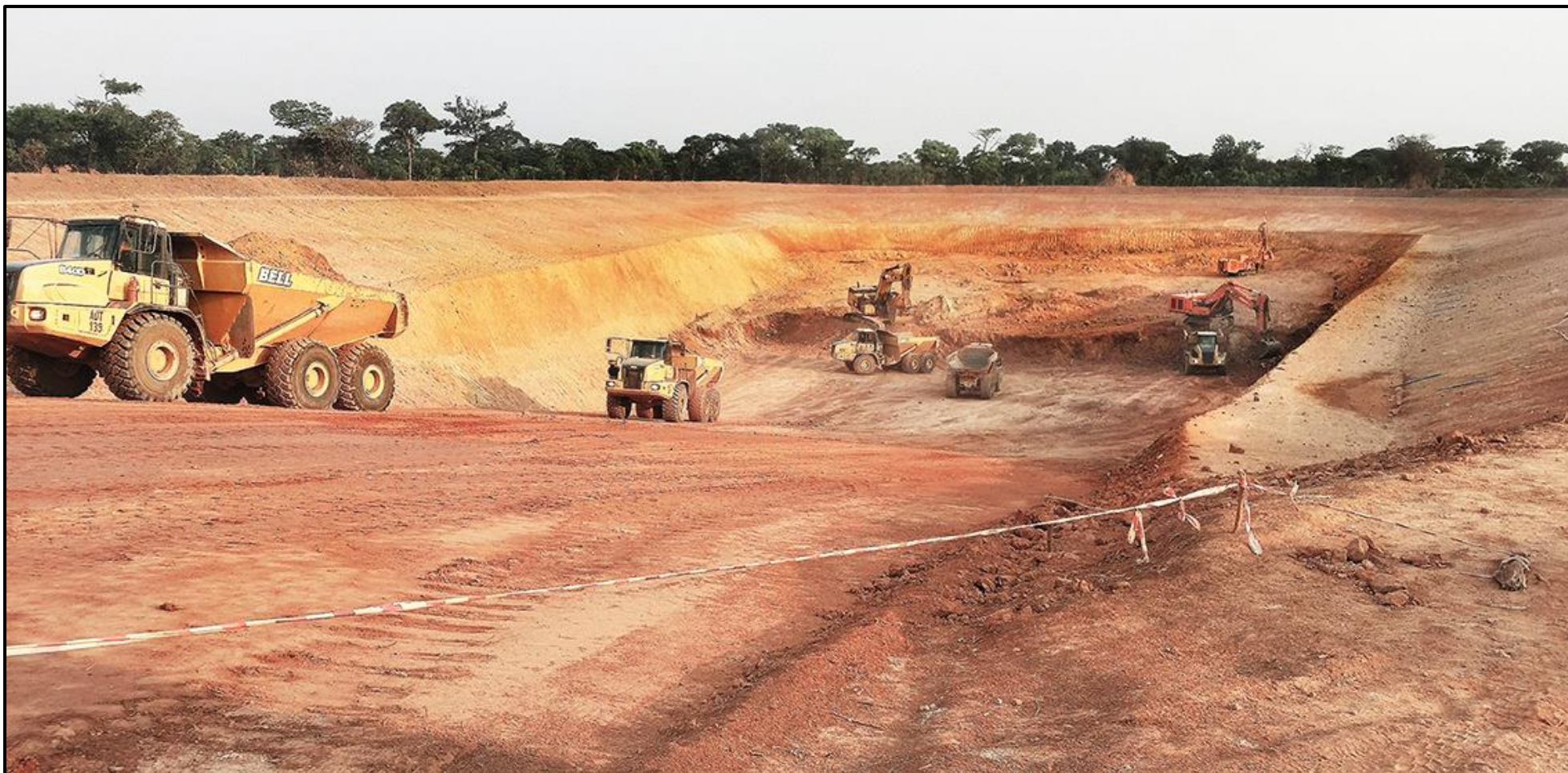
Figure 4: Box-cut excavation work, September 23, 2014.
