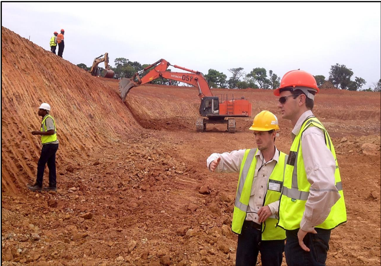
Figure 2: Ivanhoe's geologists examine progress at the Kamoa box cut, September 15, 2014.
