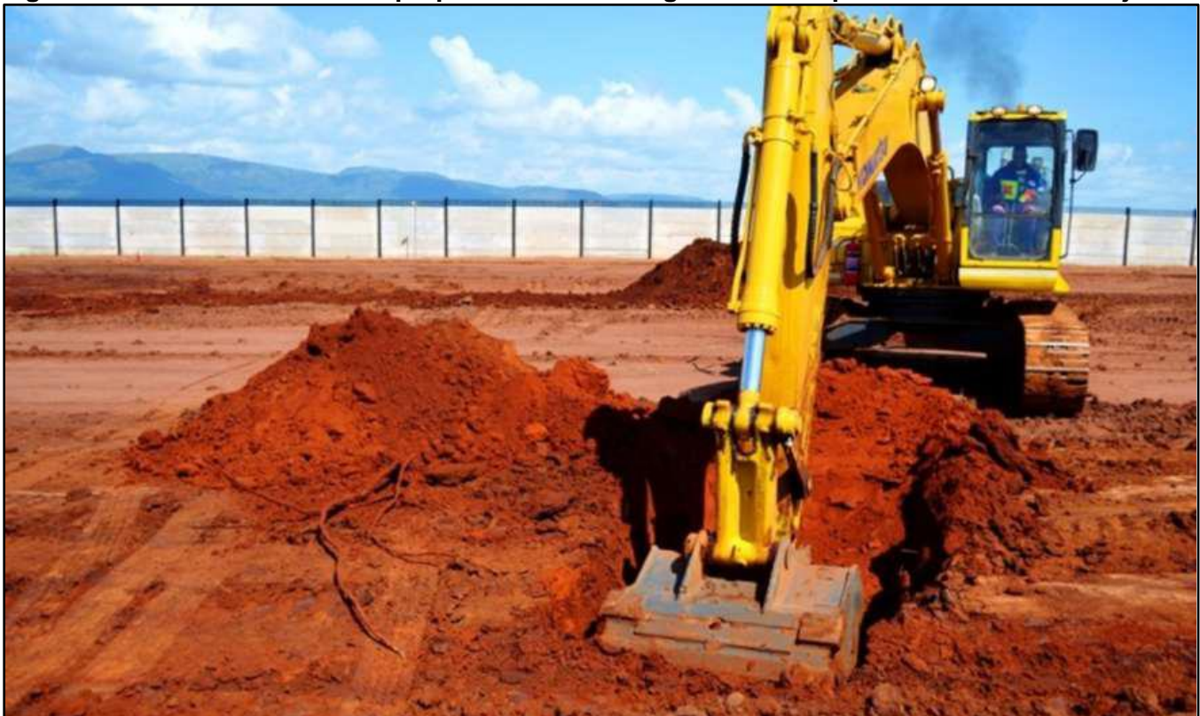
Figure 2: Box-cut excavation in preparation for sinking of bulk-sample shaft at Platreef Project.
