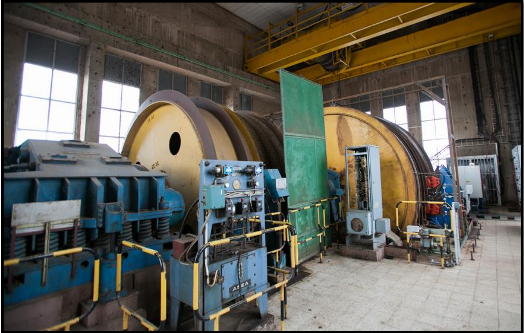
Figure 4: Ongoing refurbishment of Shaft 5 components.
