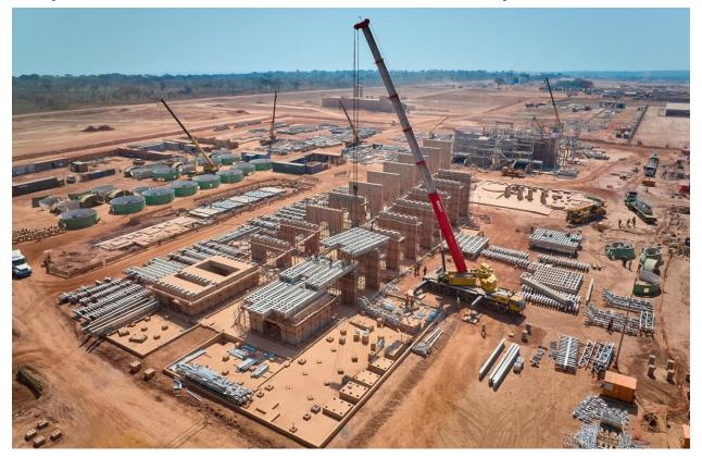
Construction of the concentrate thickener base is progressing well at Kamoa-Kakula's Phase 3 concentrator site.
