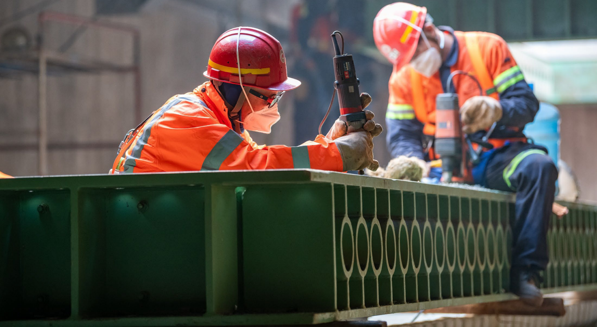
Surface crews erect steelwork at the Phase 3 run-of-mine stockpile apron feeder.
