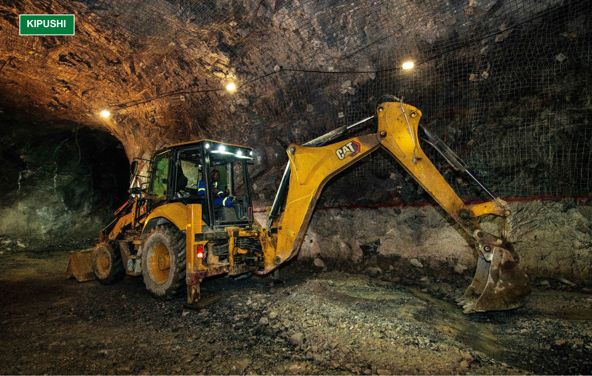
Mining personnel conducting road maintenance operations underground at Kipushi.
