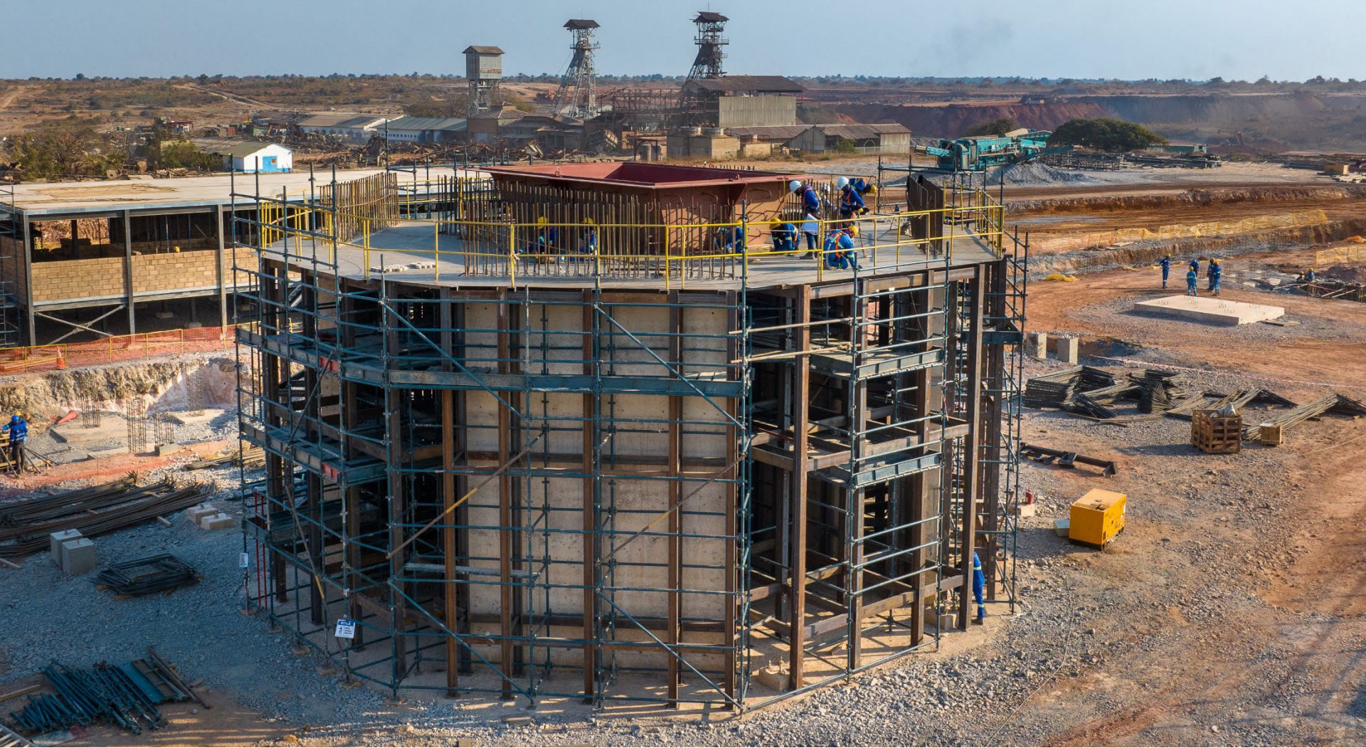
Installation of Kipushi's dense media separation feed bin is advancing well.
