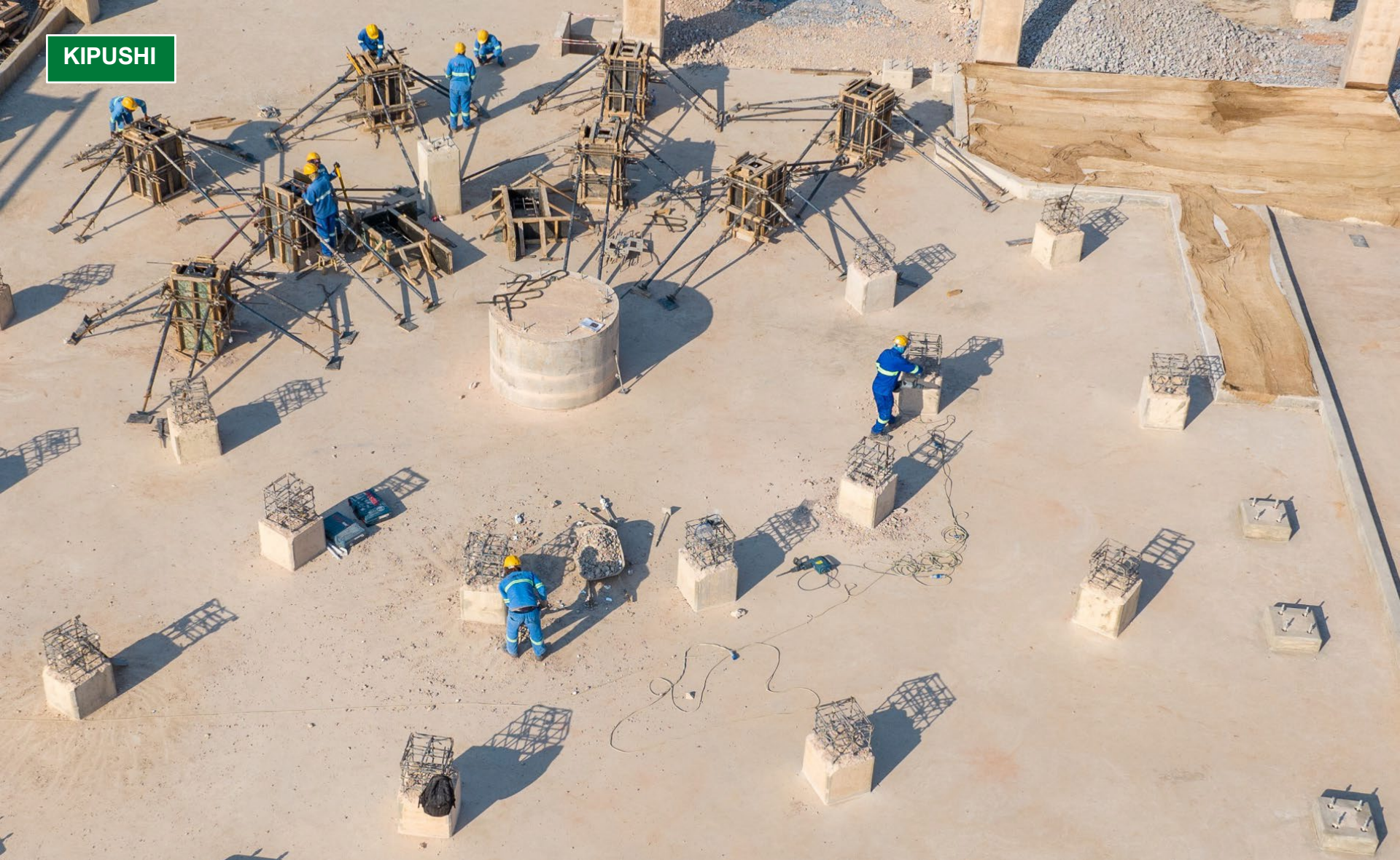
Final concrete shutter work in progress for Kipushi's flotation tails thickener.
