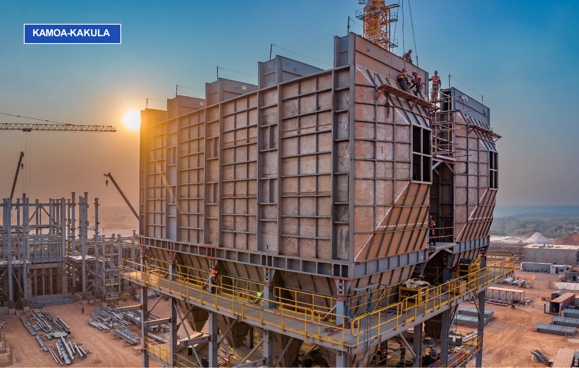
On-going construction of Kamoa-Kakula's direct-to-blister furnace off-gas handling structure.
