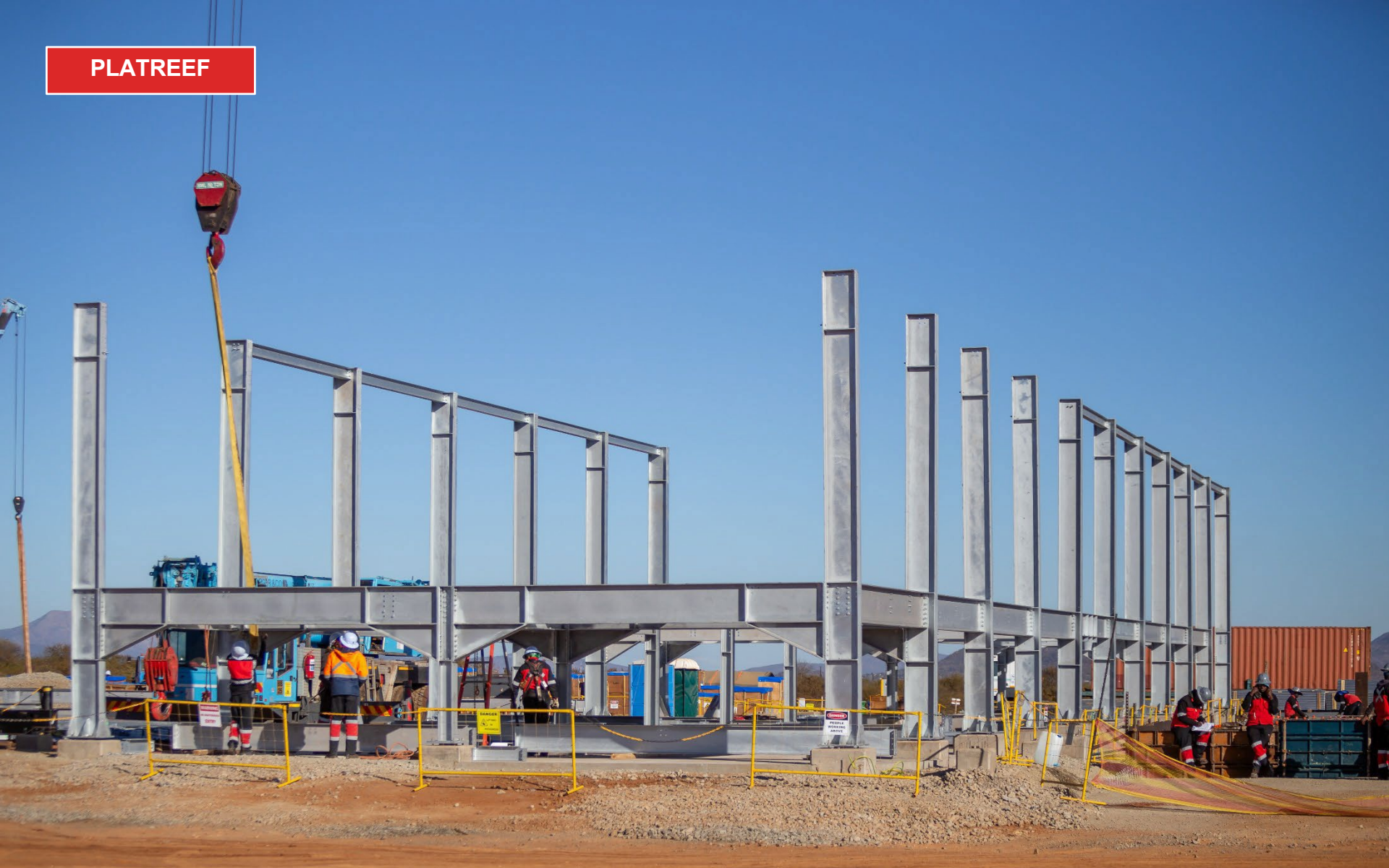
Pre-assembly and erection of steelwork advances at Platreef's plant consumer substation.
