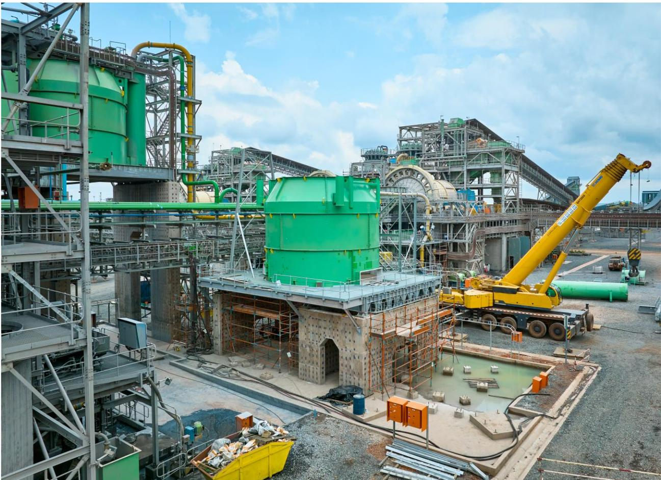
Construction of the additional concentrate thickener is advancing well. The debottlenecking program is approximately 70% complete and is tracking ahead of schedule.
