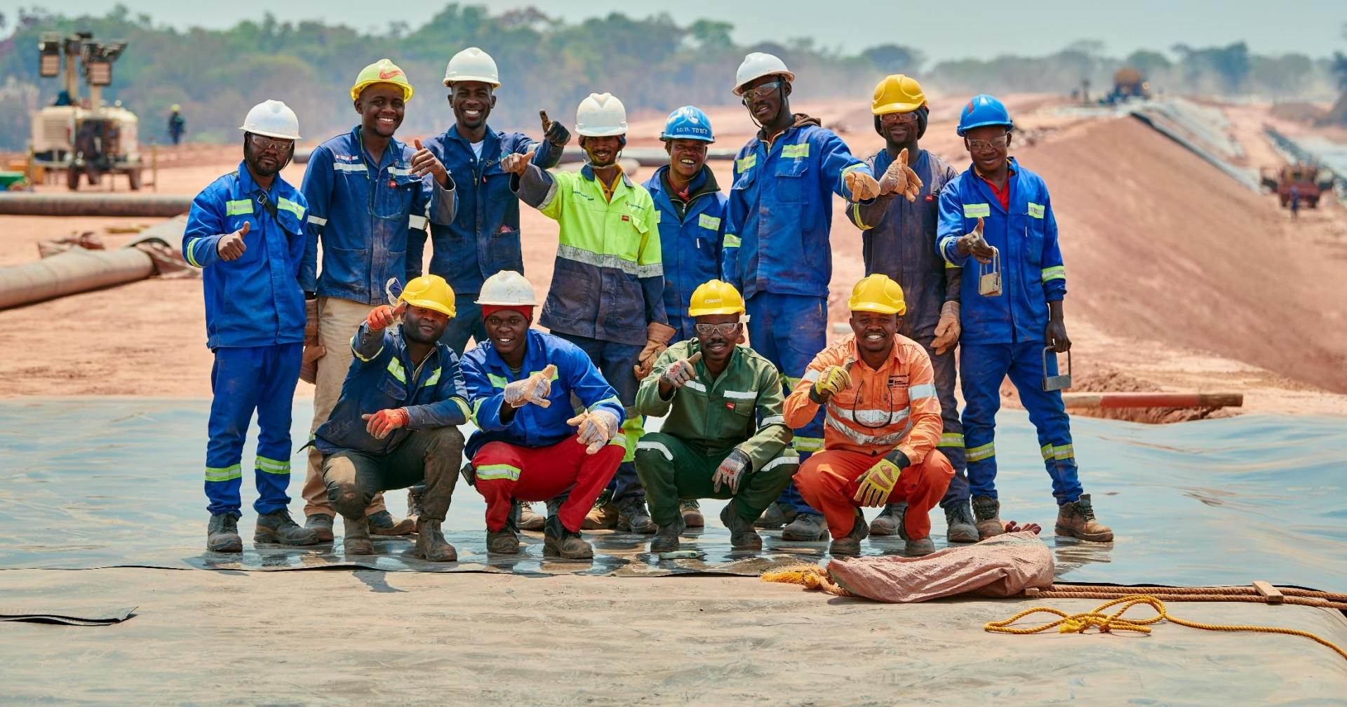
Surface construction crews at work on Kamoakakula's tailings dam expansion.
