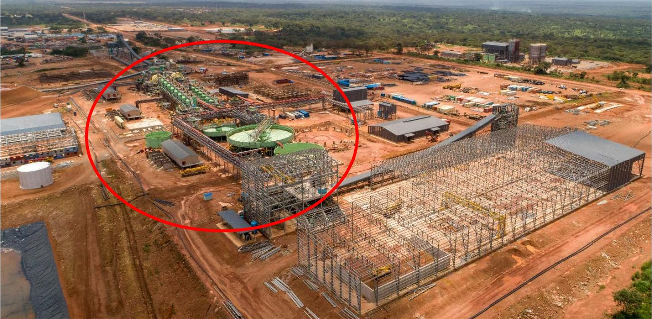
**Second stage (C2) commissioning at Kamoakakula's Phase 1 ball mills (in yellow) and the concrete foundations for the second set of ball mills for the Phase 2 concentrator (foreground), are underway.**
