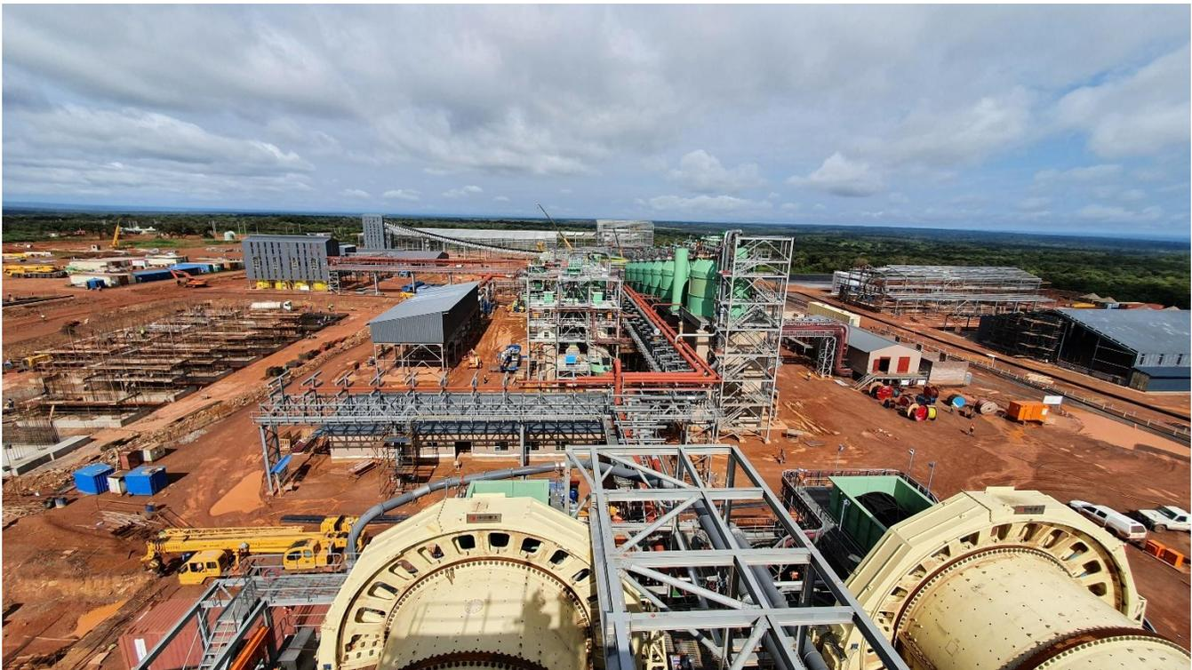
**Kakula's Phase 1 backfill plant is nearing completion. Approximately one half of the mine's tailings will be sent back underground as paste backfill to help support mined-out areas.**
