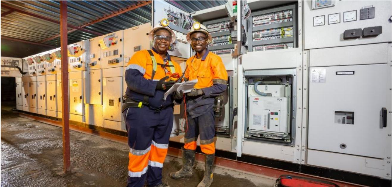
**Prince Kaomba, Electrician (left), and Paul Dikwenda, Mining Manager (right), inspecting diagrams of the 17.5-megawatt variable speed drives for the five high-volume water pumps installed on Kipushi's 1,200-metre level.**
