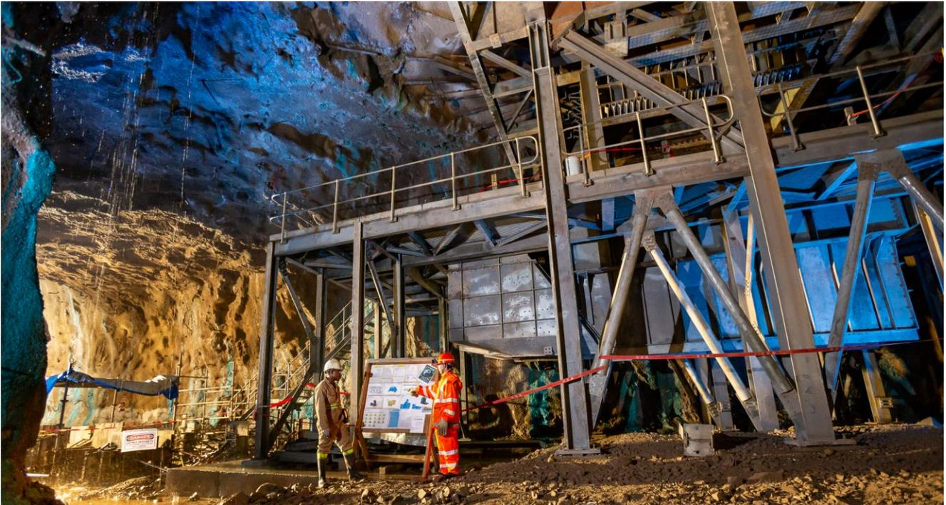
**High-volume ducts delivering fresh air to Kakula's underground workings through the 5.5-metre diameter Vent Shaft #1, allowing for an increase in the number of mine development crews.**
