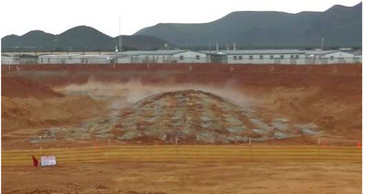
First blast at the Shaft 2 box cut.
