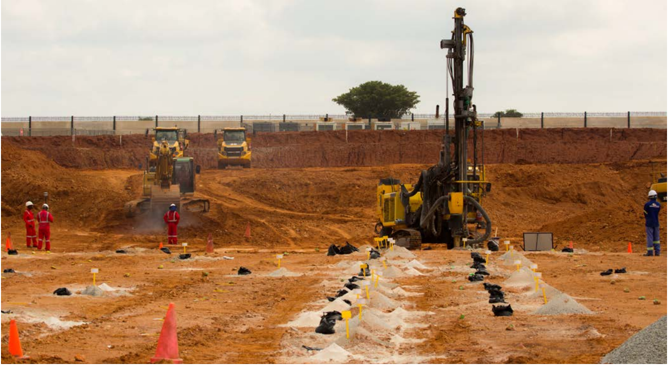
Drilling holes in preparation for the first blast at the Shaft 2 box cut.
