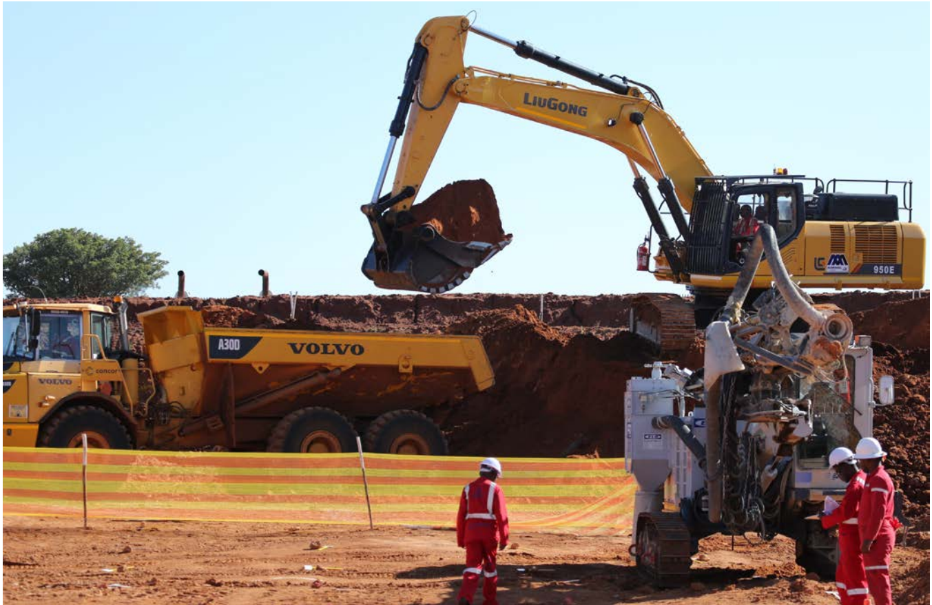
Removal of surface material during construction of the Shaft 2 box cut.
