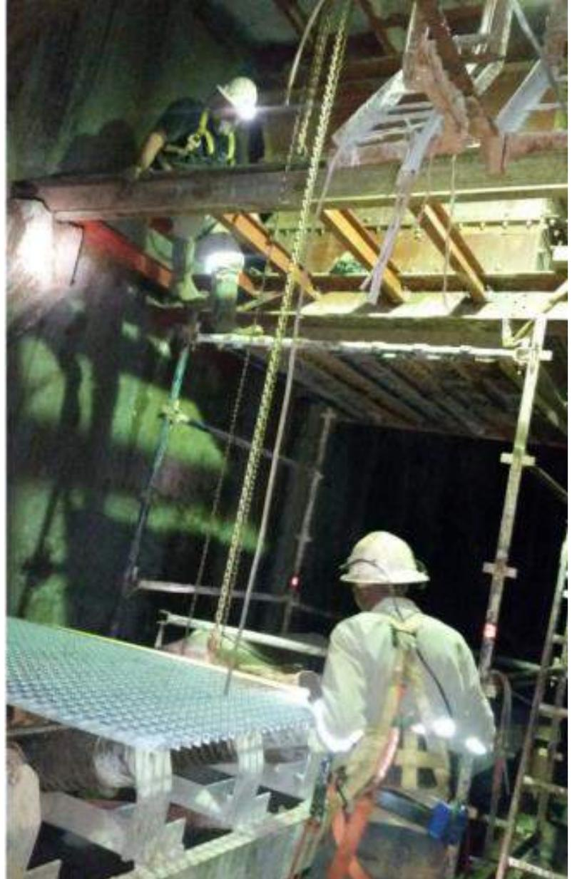
Maintenance and engineering team members installing a new platform at the mine's T2 loading area – part of the underground conveyor system.
