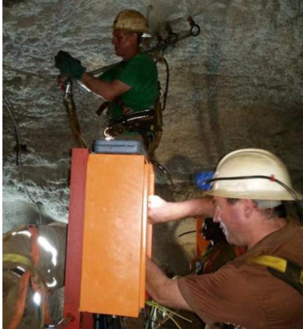
Members of Kipushi's maintenance and engineering team installing an overhead crane that was recovered from the earlier plant.
