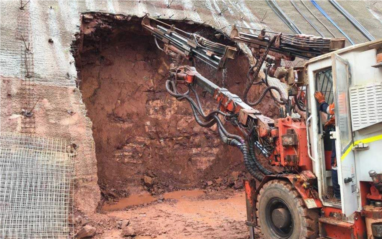
Drilling support holes for Kakula service decline following the first blast.
