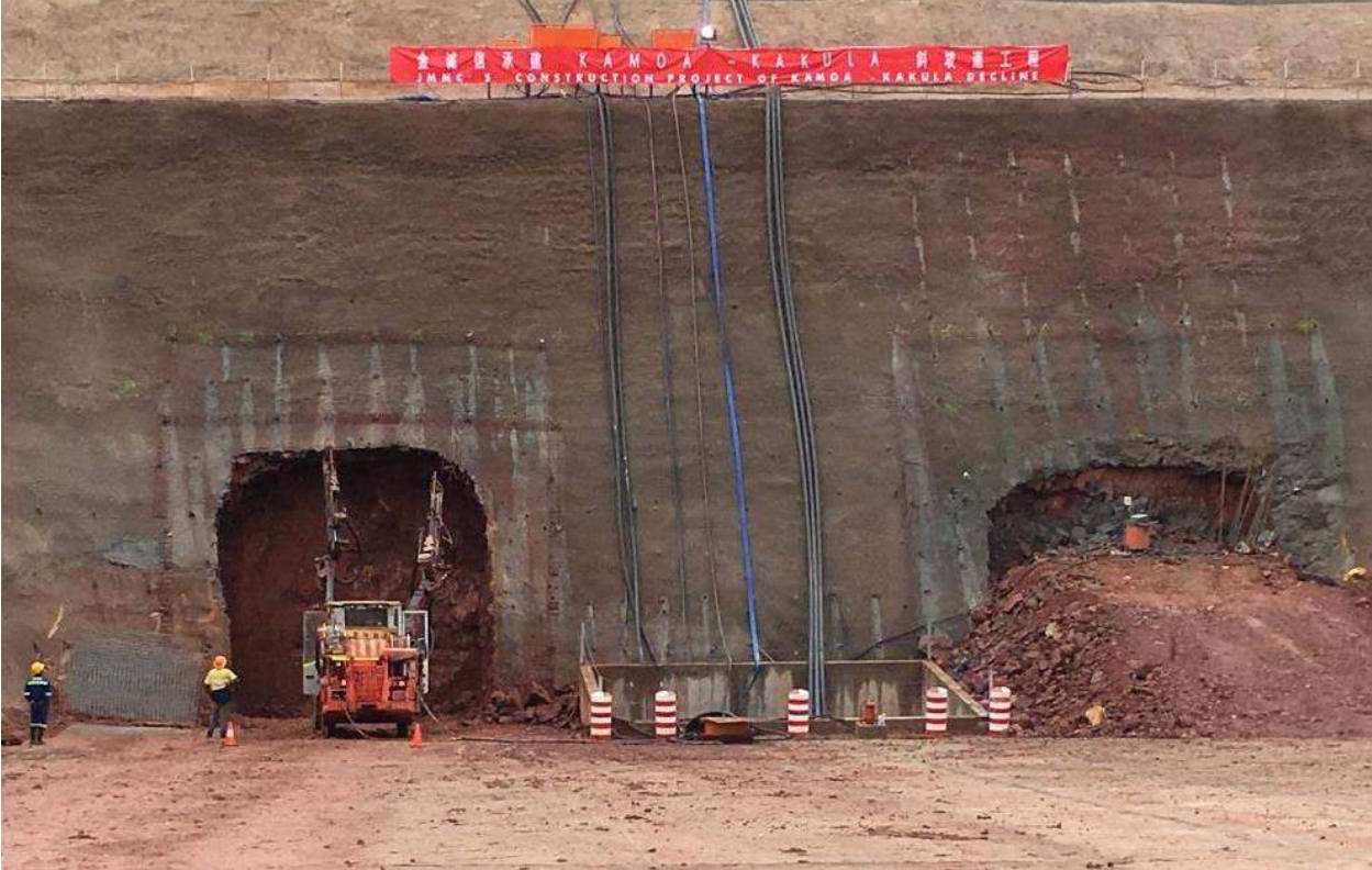
Drilling support holes for the Kakula service decline – November 17, 2017.
