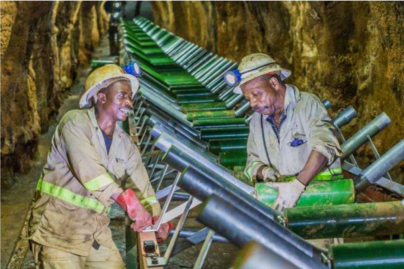
Figures 6 and 7: Installation of conveyor belt rollers in Shaft 5 ore load-out system.
