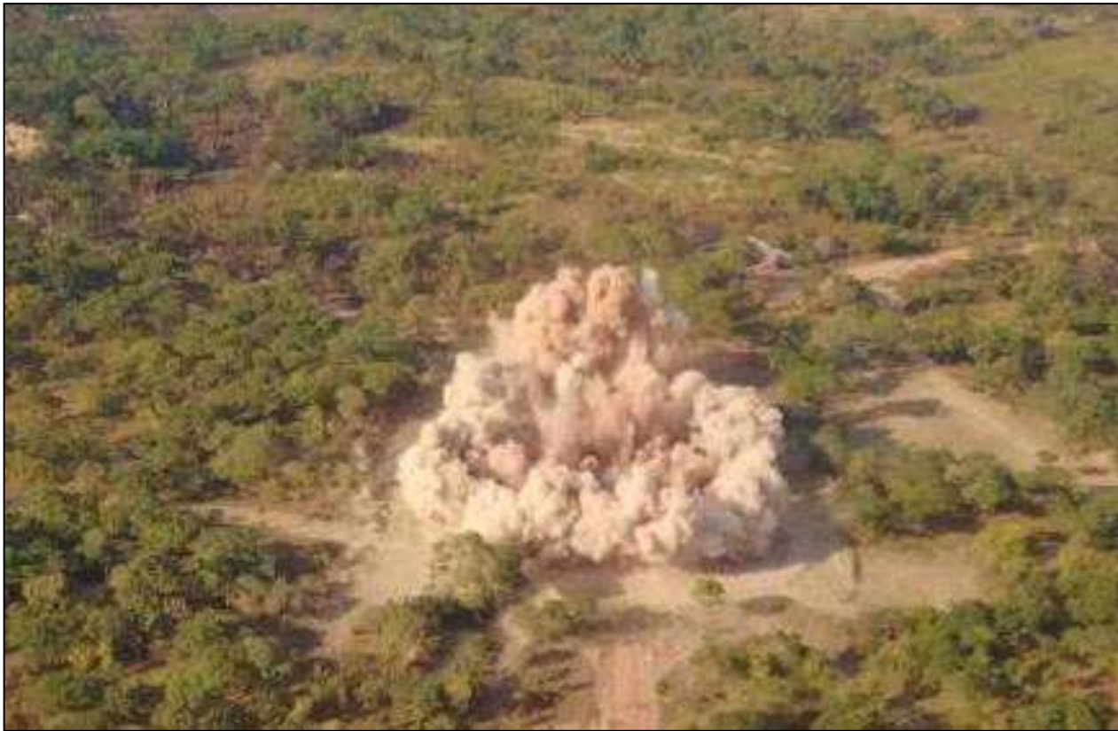
Figures 11 and 12: The first blast, followed by ongoing excavation work at the Kakula box cut.
